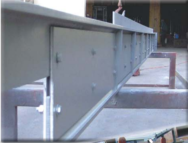
WIND BRACING SUPPORT STEEL UVA ARENA, CHARLOTTESVILLE, VIRGINIA
